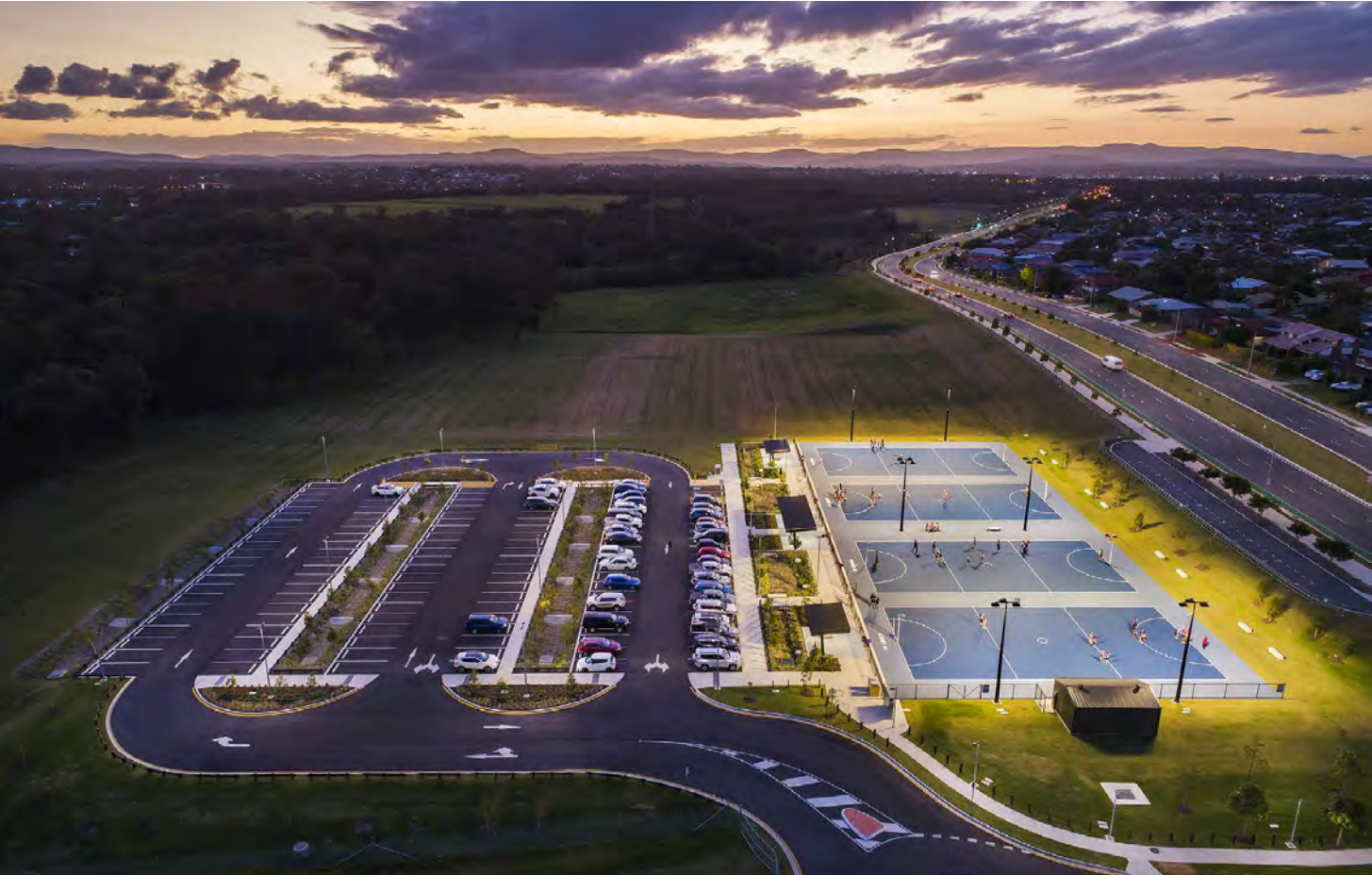
RISERVA BILL BROWN Brisbane, Australia, 2020 F-System, R-System
